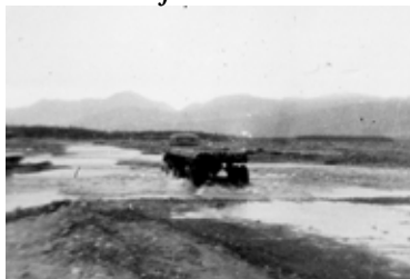
#99: Hauling pipe north
