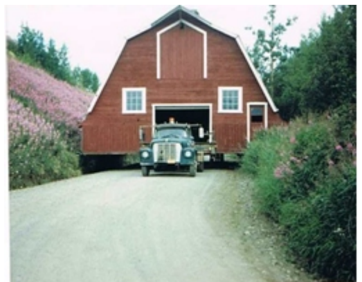
Moving the McCombs/Johan Johnson Colony Barn along Fairview Loop Rd.
